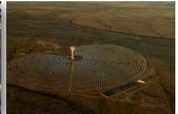
Solar thermal power plant
