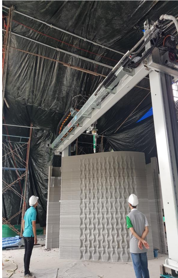
CNC Design VSF Concrete Onsite Printer for SCG Thailand
