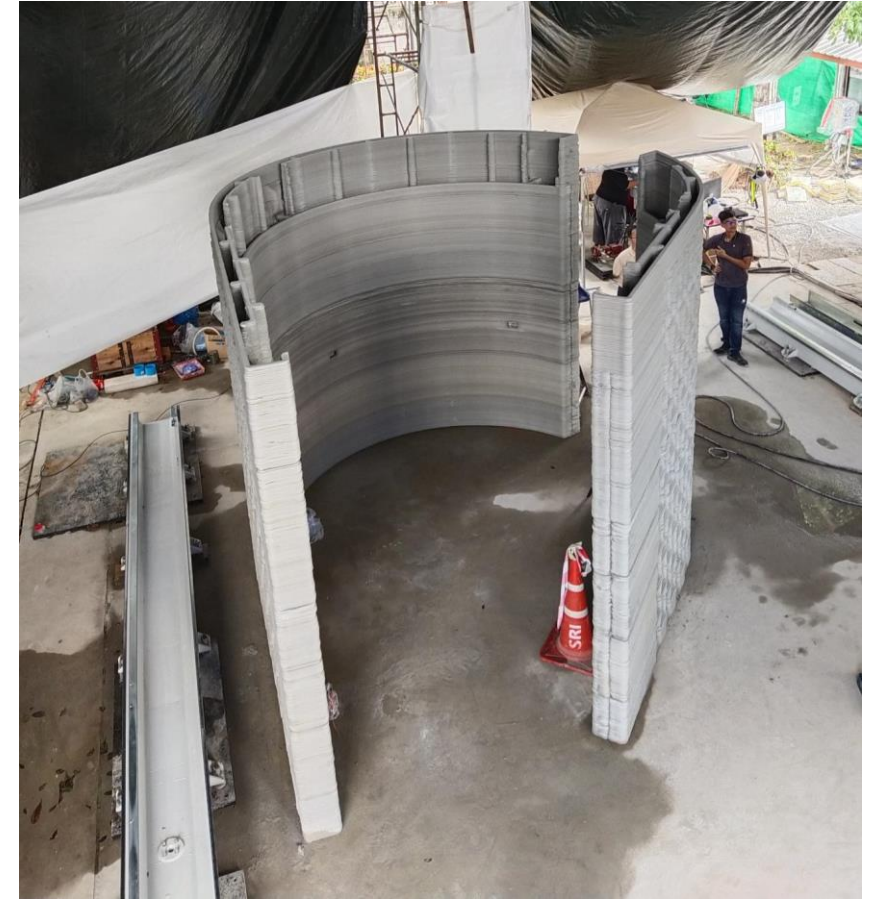
CNC Design VSF Concrete Onsite Printer for SCG Thailand
